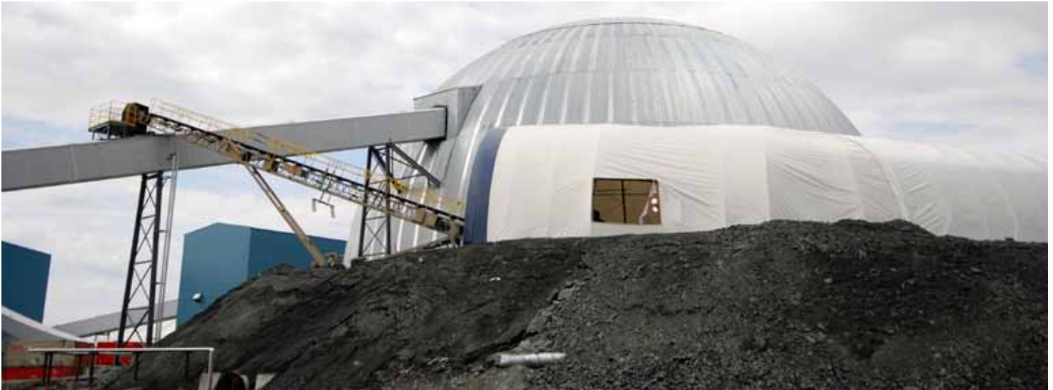
UP NORTH: The massive ore storage dome at gold mining firm Agnico-Eagle's Meadowbank mine in Nunavut. To date, it is the only mine working in Nunavut and it has cost the company a total of $1.5 billion so far. REUTERS/EUAN ROCHA
