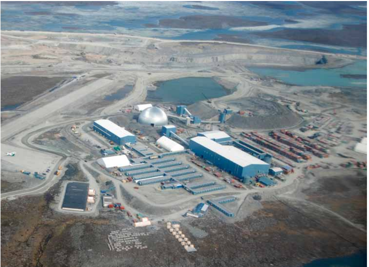
An aerial view of Agnico-Eagle's Meadowbank mine and processing facilities in Nunavut, Canada photographed on June 28, 2011. REUTERS/EUAN ROCHA
